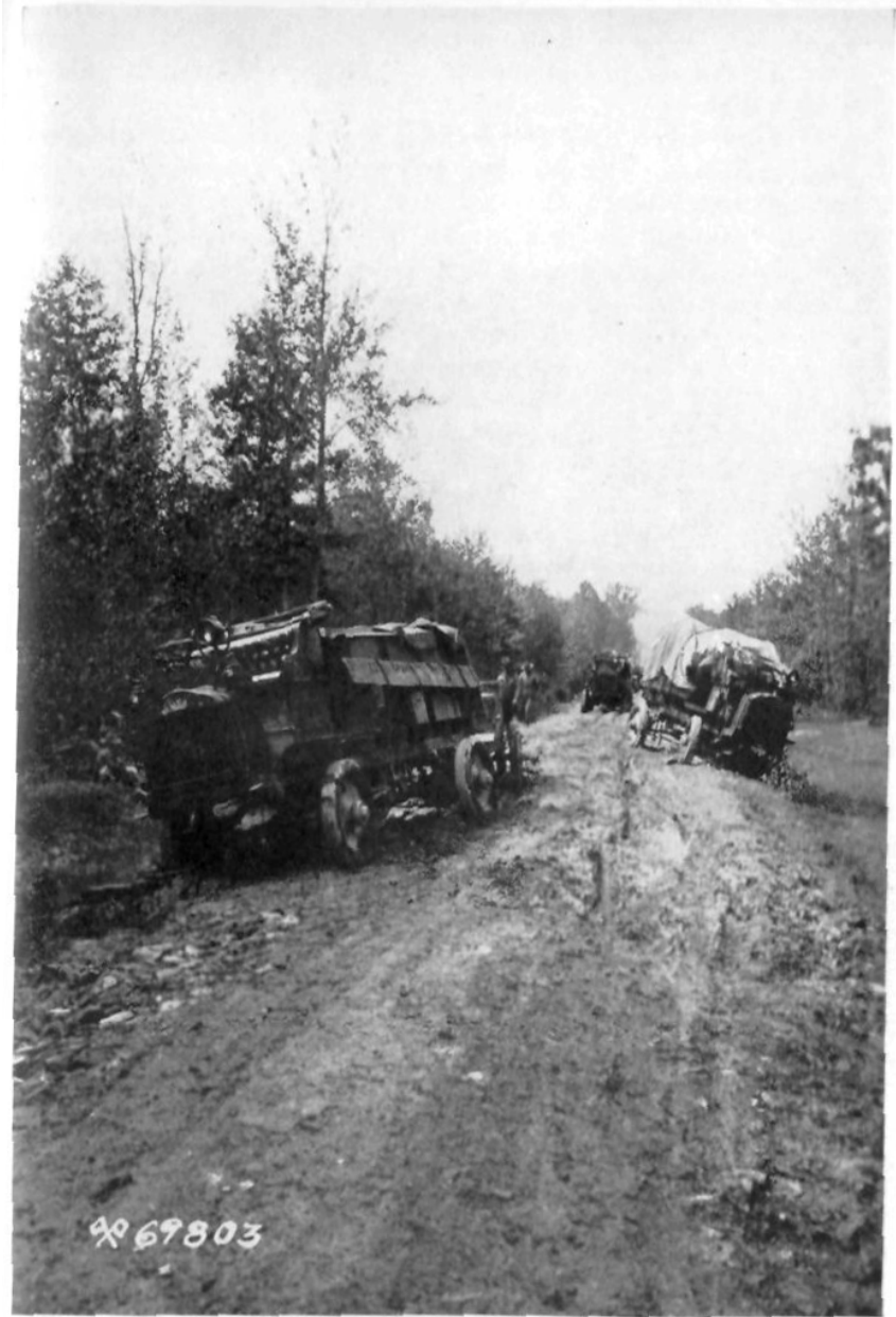
PHOTOGRAPH No. 3.—TRUCKS STALLED FOR LACK OF CHAINS. VERY SLIPPERY CLAY ROAD. QUITE HIGHLY CROWNED.
